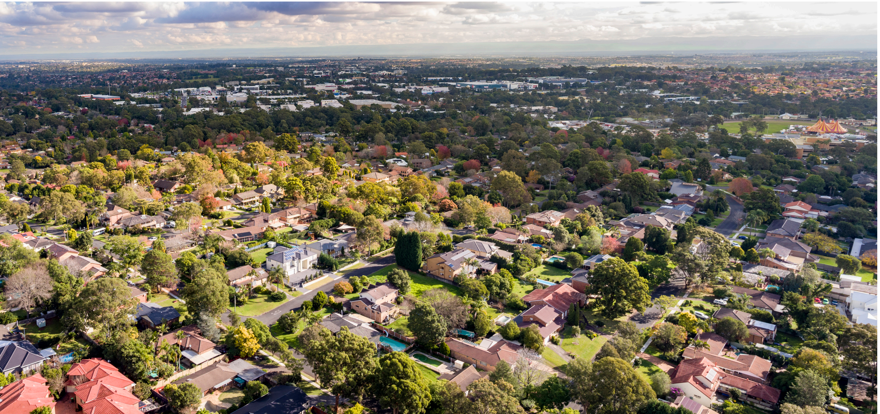
AERIAL VIEW OF EXISTING AREA
